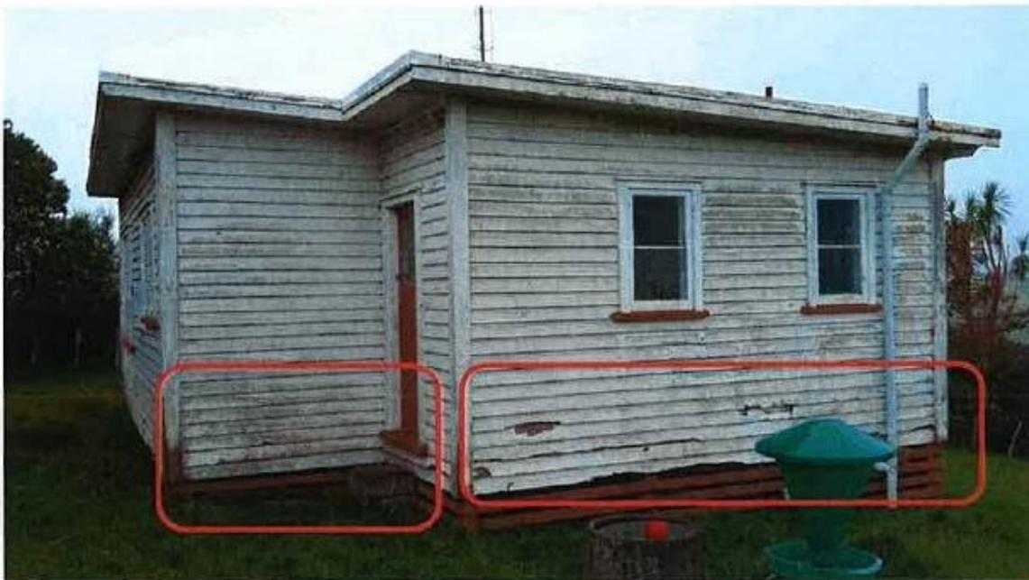
1. Front and side elevation showing rotten cladding and paint system failure.
