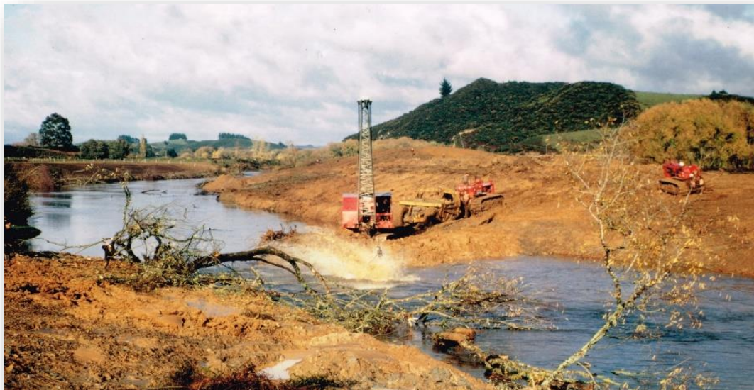
ŌTOROHANGA STOPBANK CONSTRUCTION 1962
