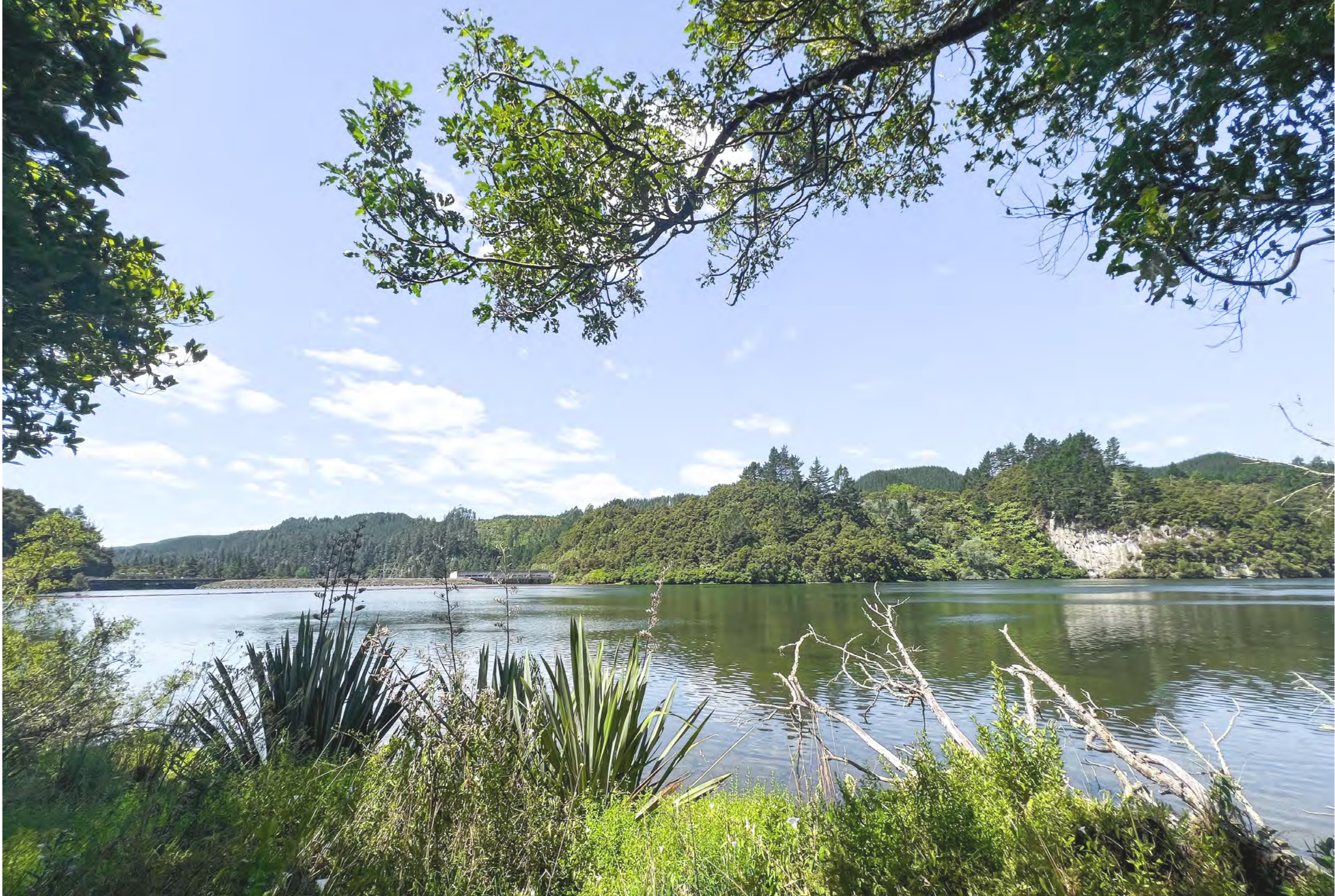
Figure 1. View of Waipapa Dam
