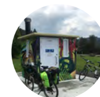
2023 - Arohena toilet (Est. 2018)
