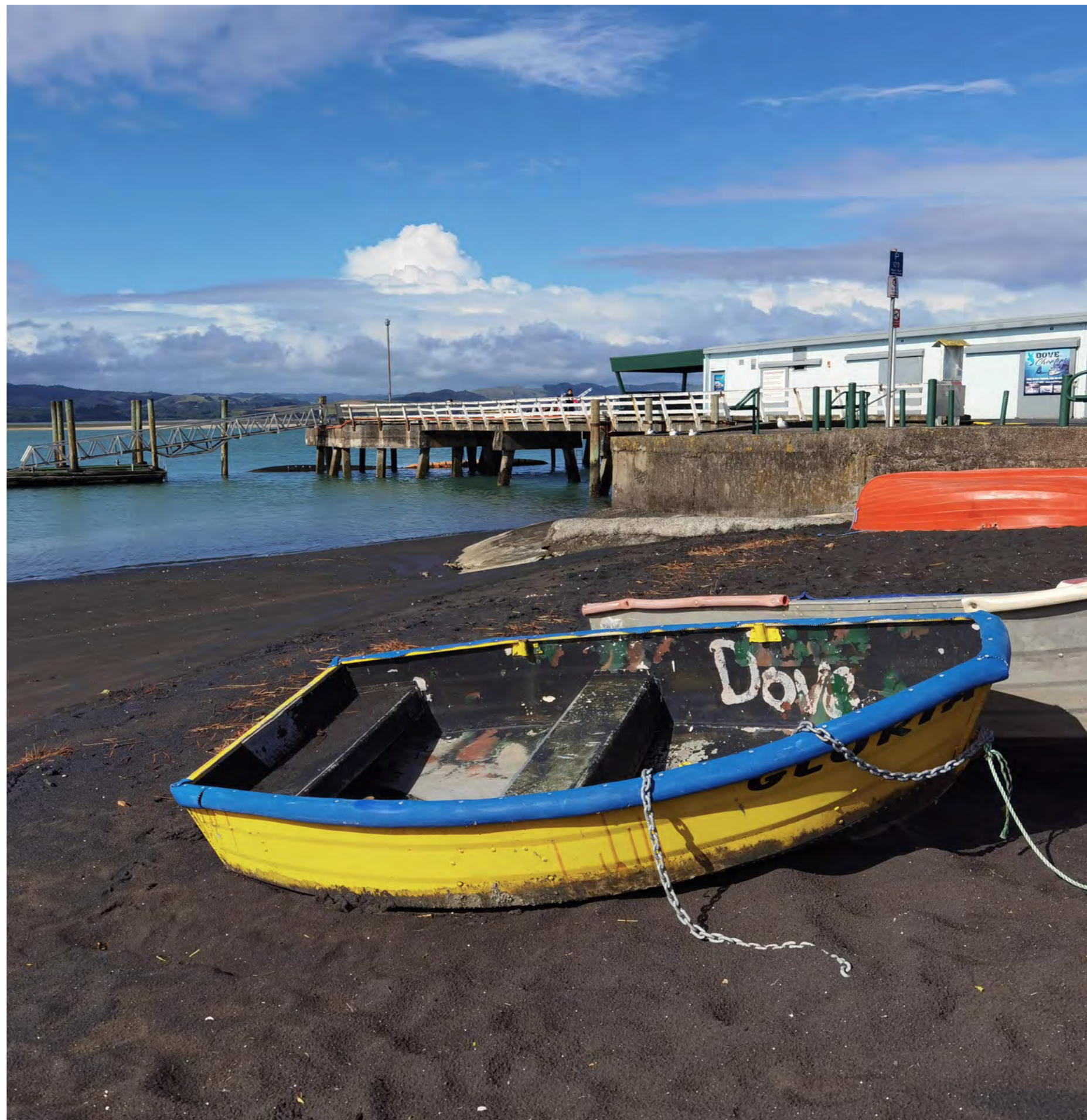
Figure 30. View of Kāwhia Wharf
