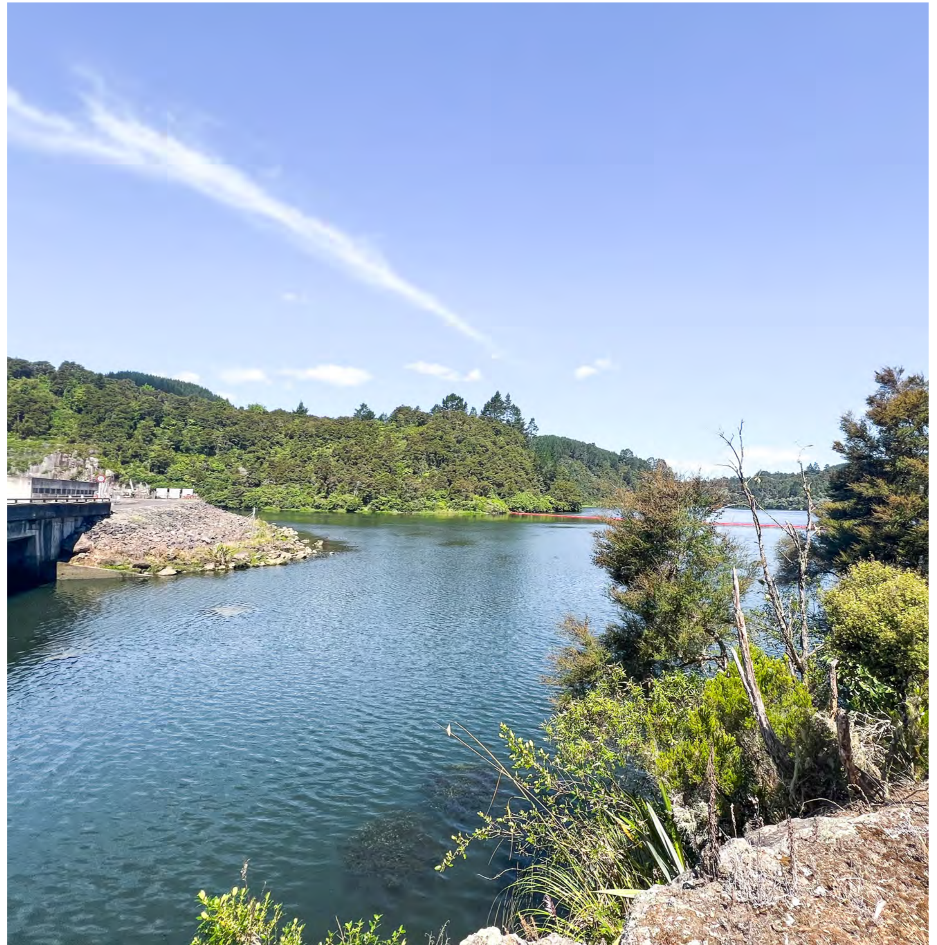
Figure 27. View of Waipapa Dam
