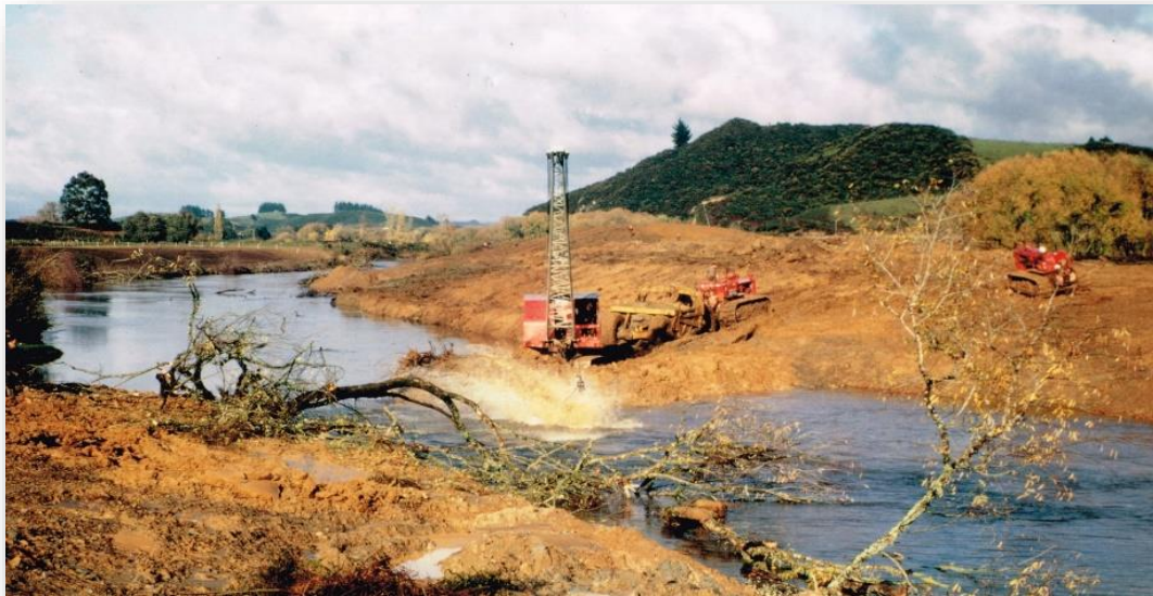
ŌTOROHANGA STOPBANK CONSTRUCTION 1962
