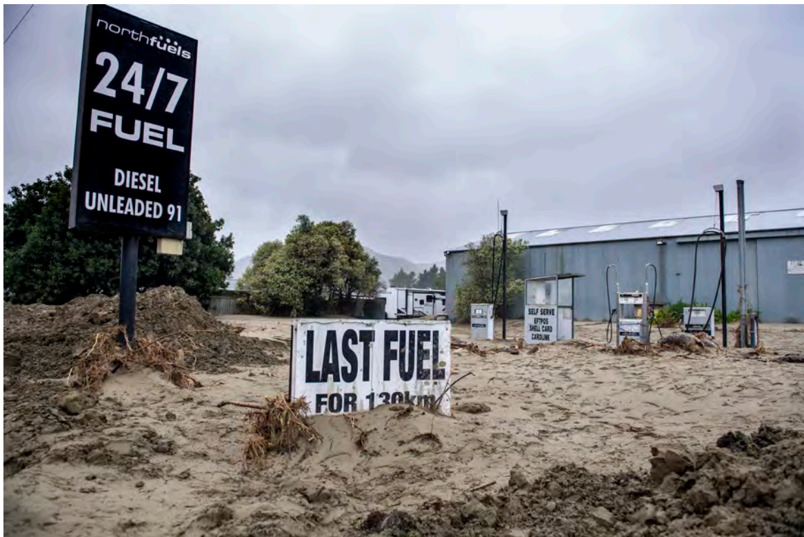
Image: Petrol station buried under silt in Esk Valley, Hawke's Bay. Source: NZDF
