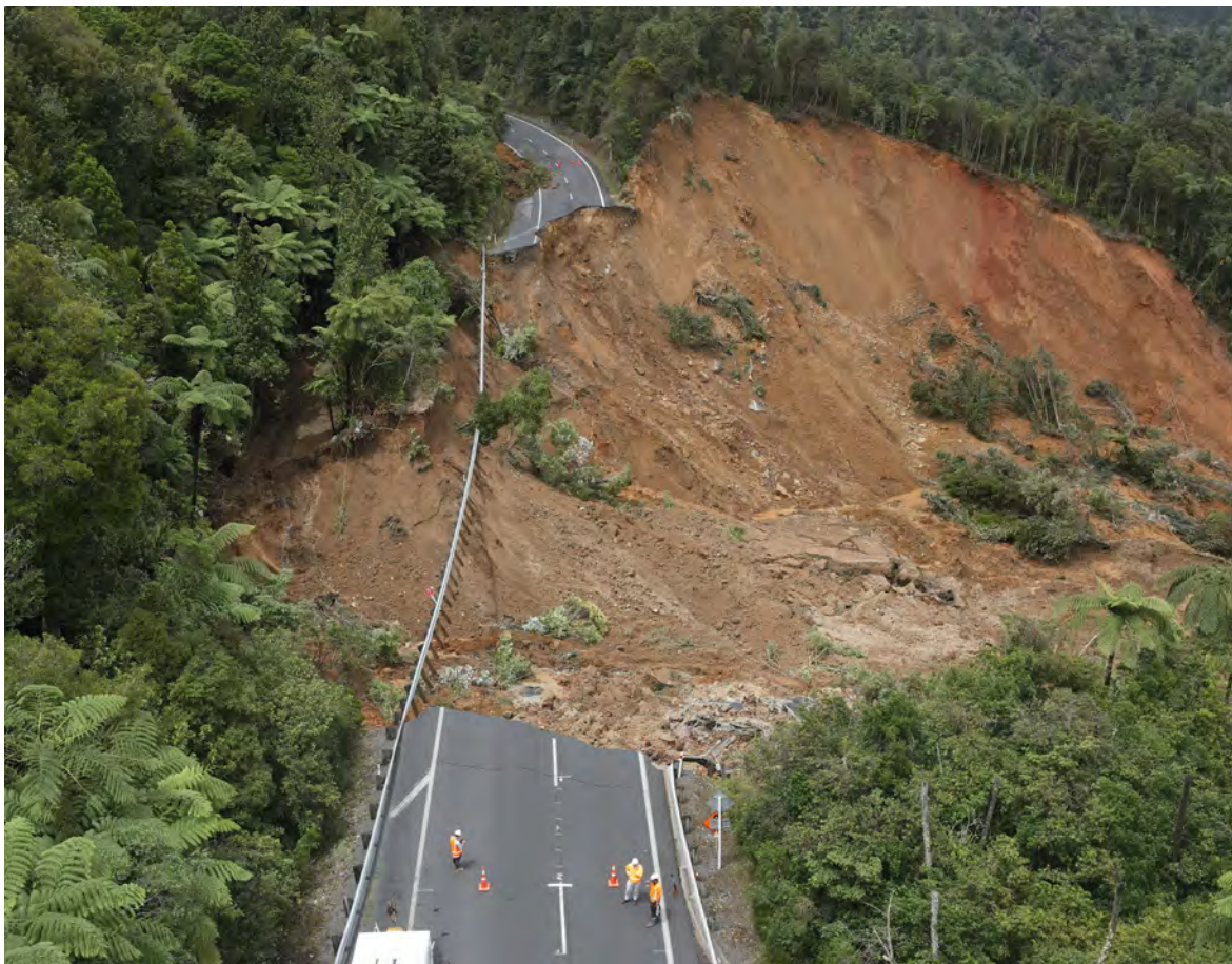
Image: A major slip on SH25. Source: NZTA
