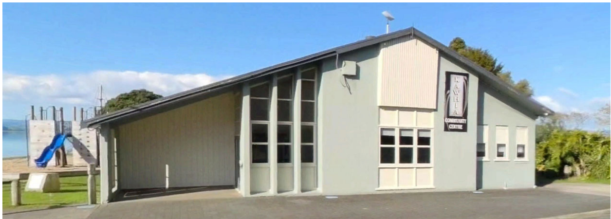
Front entrance on West side of building showing double pitch gable roof and front meeting room with projector room above and kitchen to the right and toilet area with extended lean-to roof on left side.
