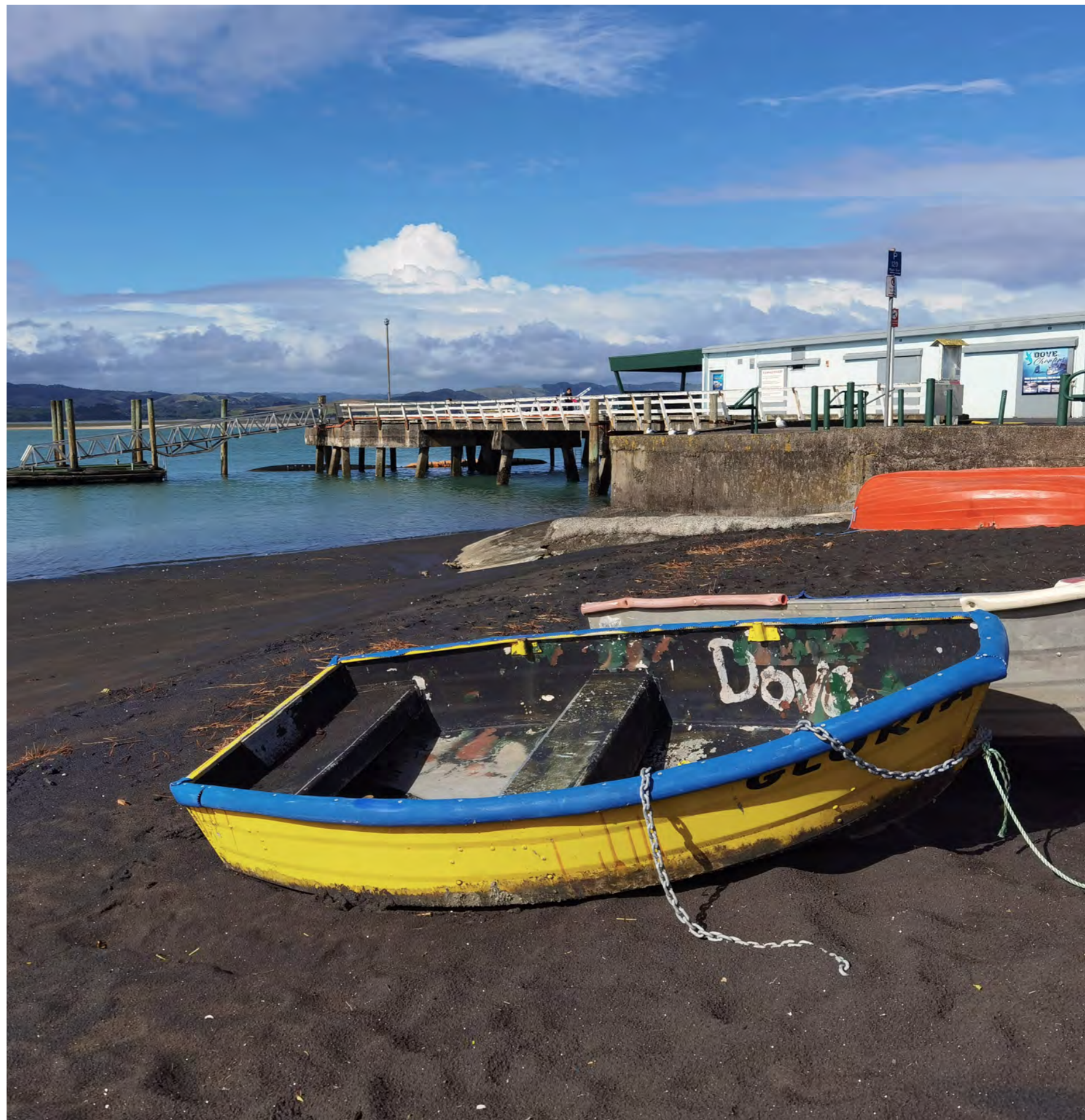
Figure 30. View of Kāwhia Wharf
