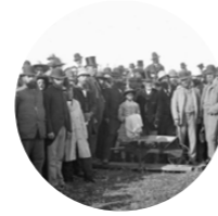
1885 - 'First sod' for the main trunk railway in Ngāti Maniapoto territory
