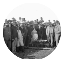
1885 - 'First sod' for the main trunk railway in Ngāti Maniapoto territory
