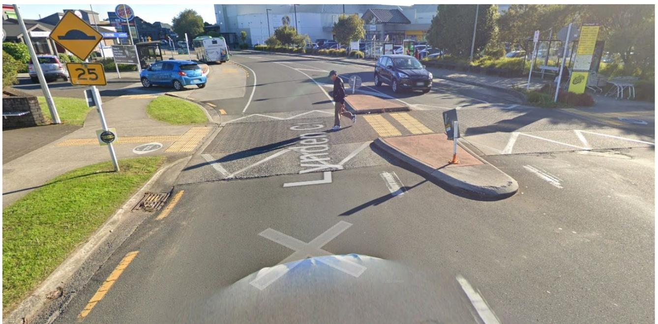
Figure 2: Typical raised pedestrian platform
